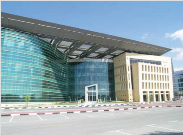
Ministry of Public Works, Al Shaafar General Cont. KEO International Consultant, Al Qusais, Dubai
