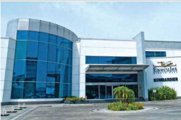
Dubai Airport Free Zone, FNC Cont., Client: Execujet,
