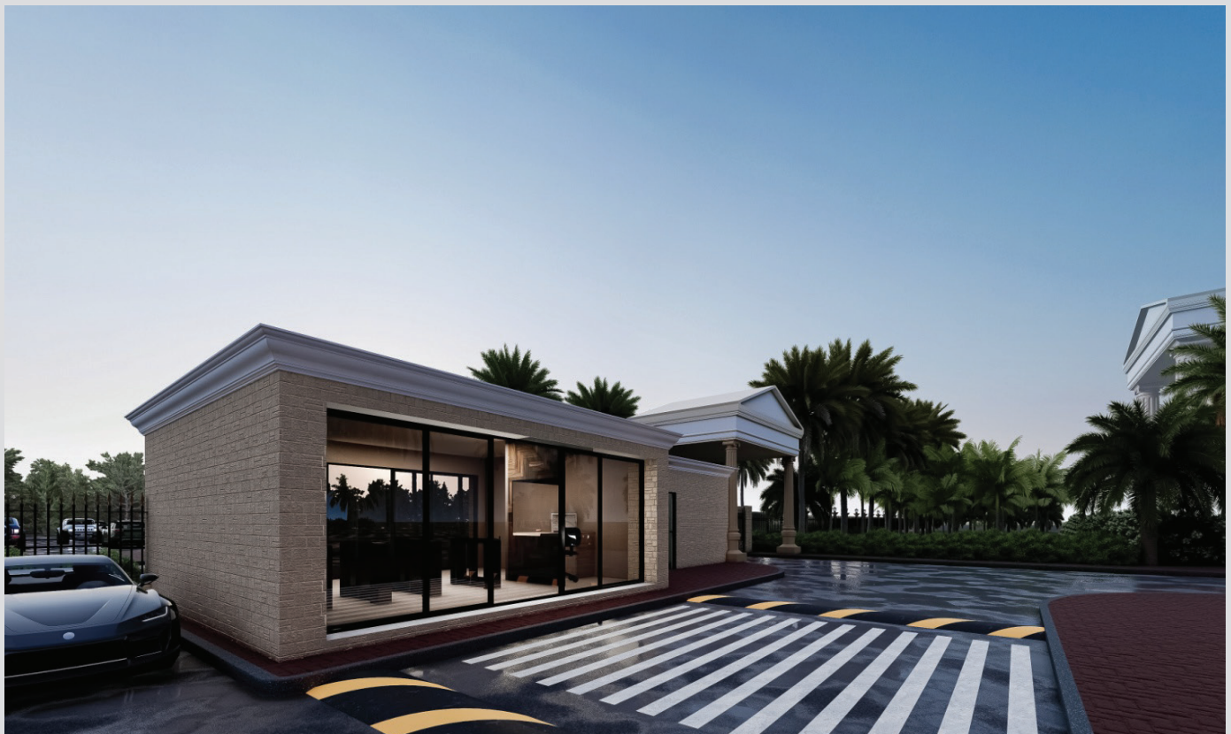
AMERICAN UNIVERSITY DUBAI (AUD) PLOT NO. 3820121 Al Safouh Second Dubai, UAE Contractor: M/s Al Tariq Contracting L.L.C Consultant: M/s Erga Progress Engineering Conlutants
